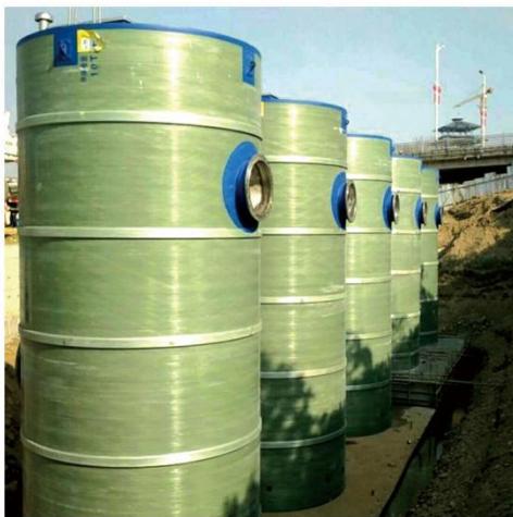
一体式玻璃钢泵站 Integrated fiberglass pump station
