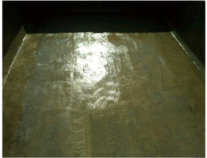
污水池防腐现场 Sewage tank corrosion field
