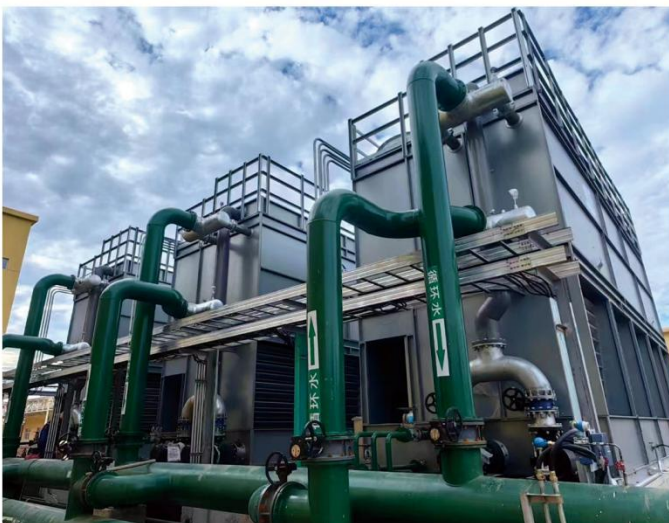
镀镁铝锌闭式冷却塔 Magnesium aluminum zinc coated closed cooling tower
