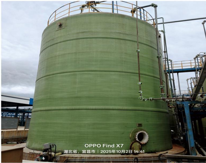
PP-FRP成品罐 PP-FRP finished tank
