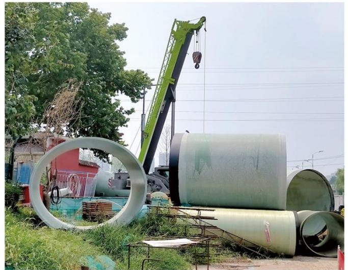
玻璃钢顶管安装 Installation of fiberglass top pipe
