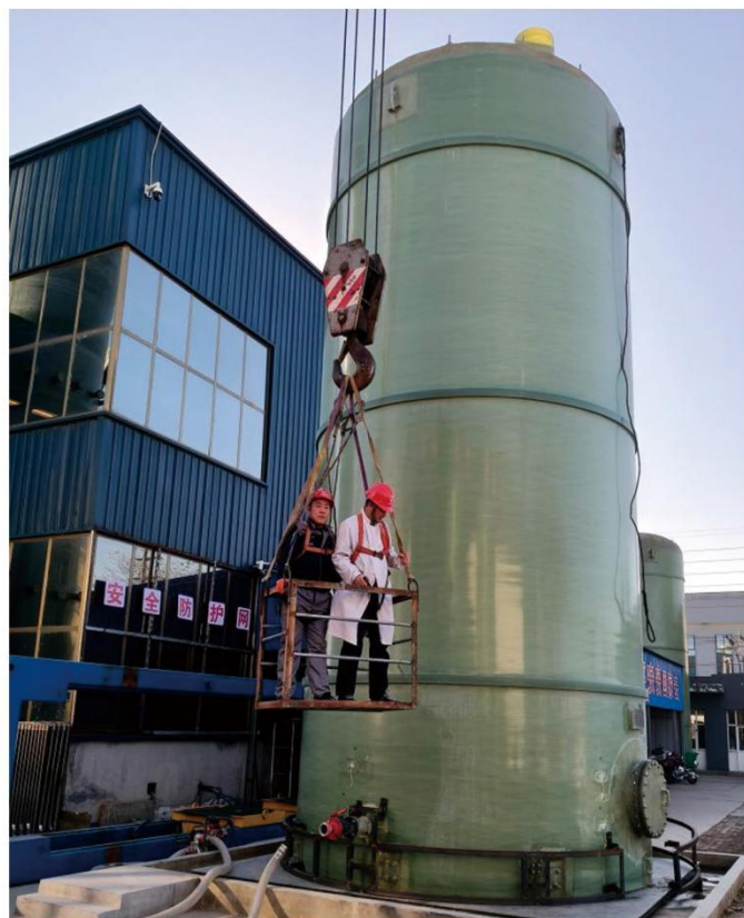
漂洗罐 Rinsing tank
