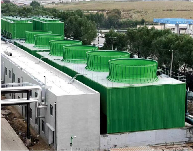
玻璃钢冷却塔 Fiberglass Square Cooling Tower
